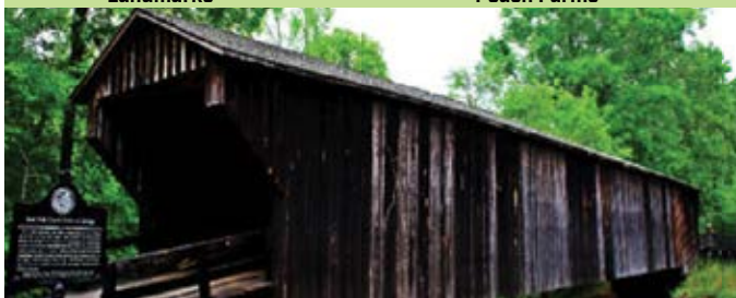
Red Oak Creek Covered Bridge
